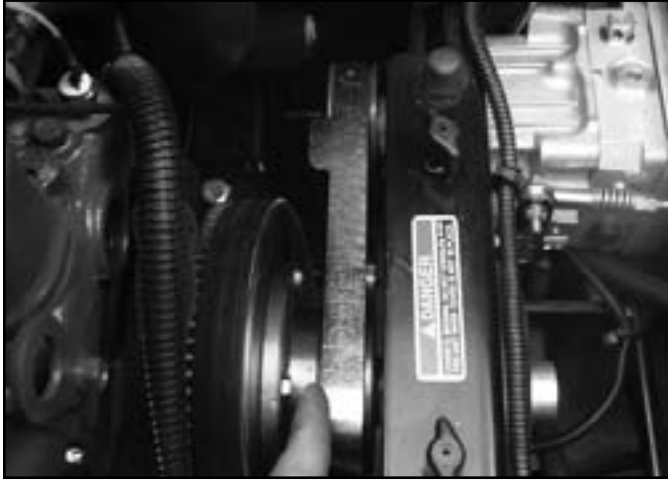
Fig 292 hydro belt alignment
